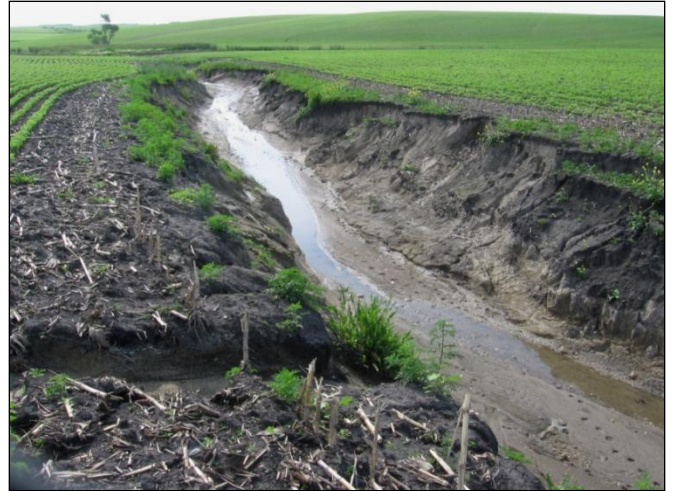
Once complete, gullies such as these will be closed and farmable.
