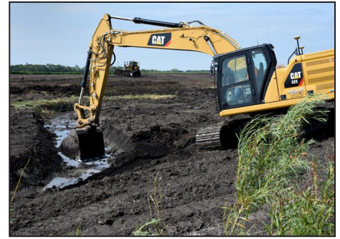
Left and right: Phase 2 of the Whiskey Creek stream restoration, seen here on Aug. 2, 2022, connected to Phase 1 work completed in fall 2021, which created 4.3 remeandered stream miles within a 3.3-mile corridor along Minnesota Highway 9 in central Wilkin County. Middle: Vegetation flourished along a segment of Whiskey Creek. Remeandering the once-straightened channel will help to slow velocity, curb bank erosion and avoid sediment build-up.
